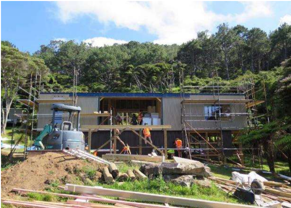
FIG 20: The new lodge takes shape November 2017. (P. Hutton).
