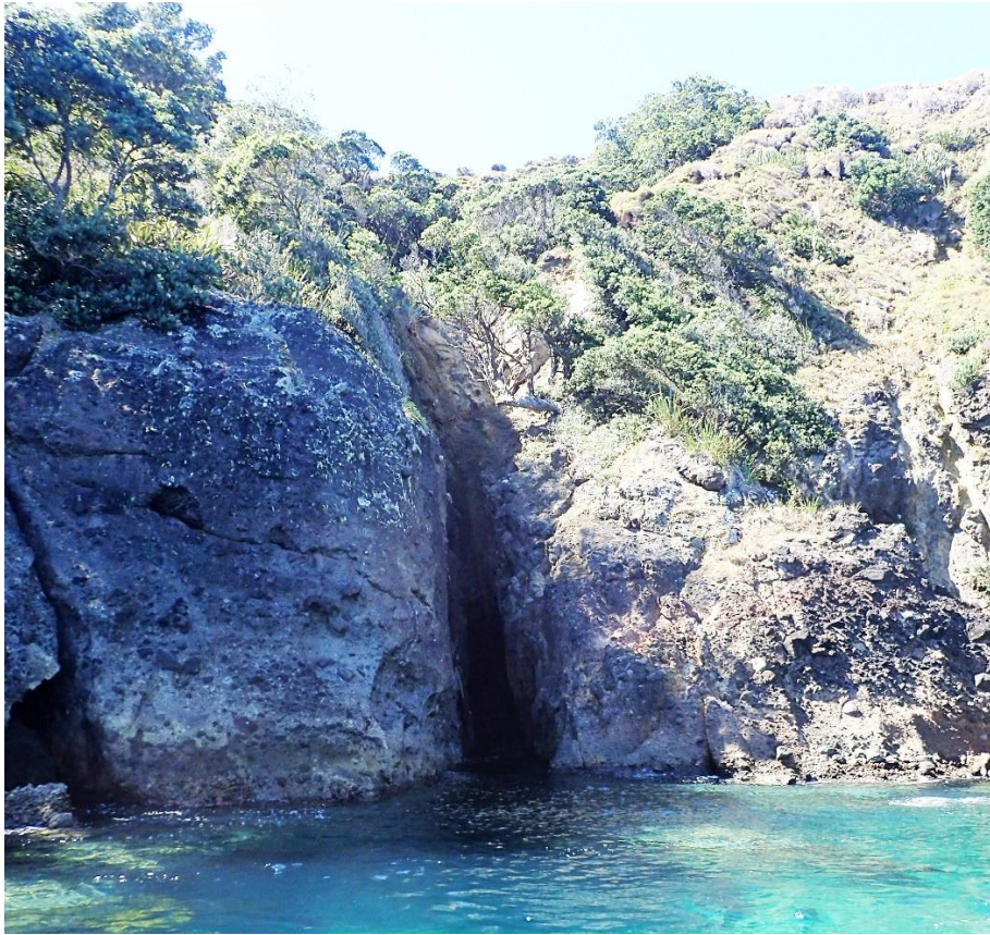
Deep incised gut along weak joint.
