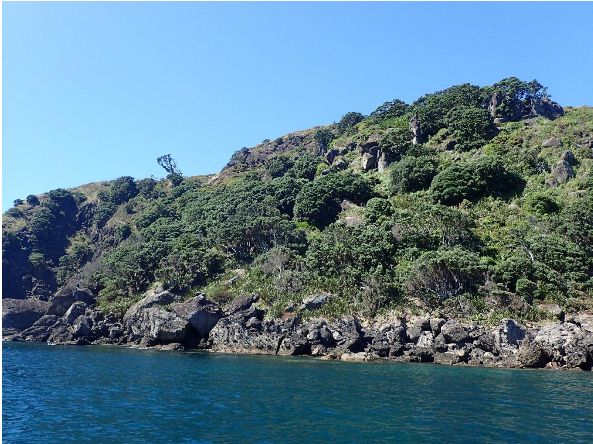
Large rock fall extends most of way up slope.
