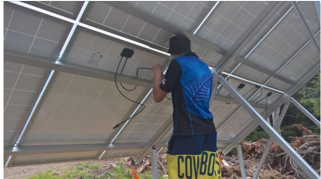
Tom wiring up the panels on the inside
