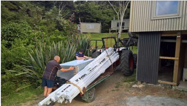
20 solar panels ready to go to the site
