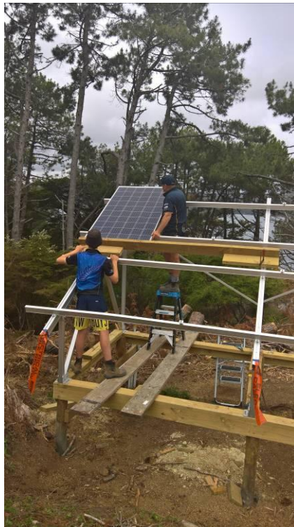
Ricky and Tom installing panels
